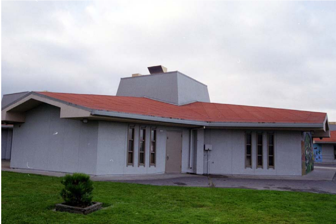
Figure 6: Classroom Building, Unit C, east face
