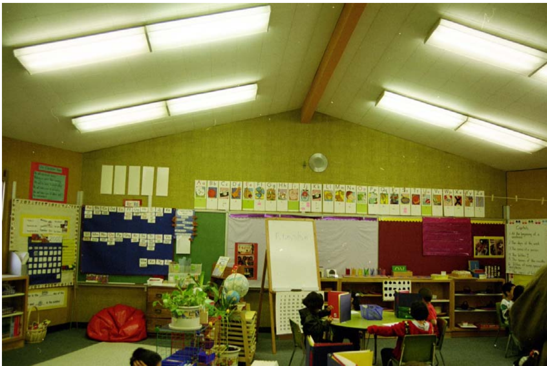
Figure 7: Classroom Buildings, Units B & C, interior
