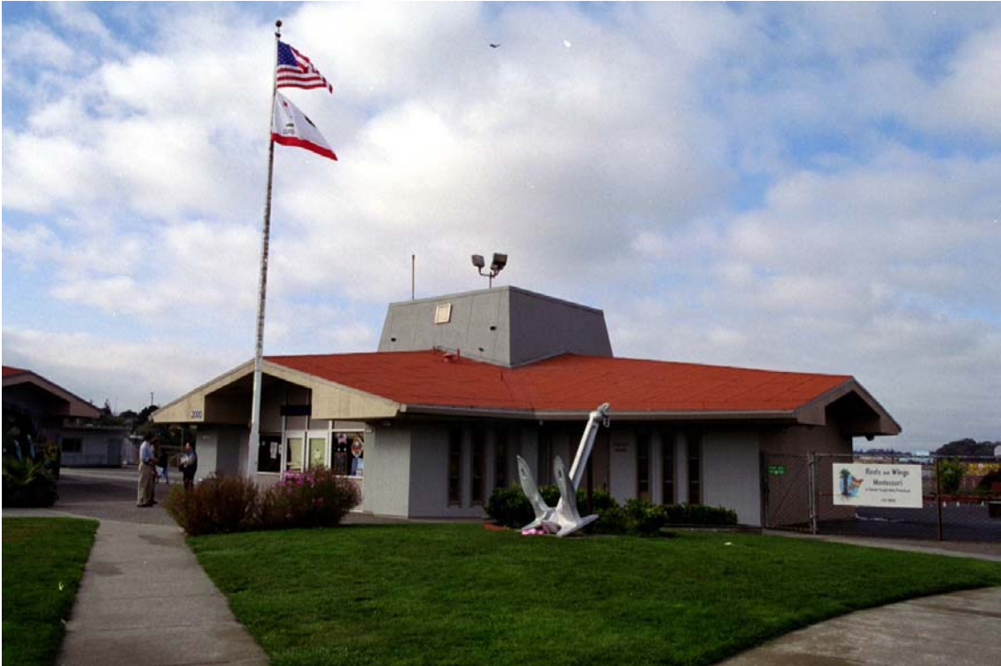
Figure 3: Administration Building, Unit A, north face
