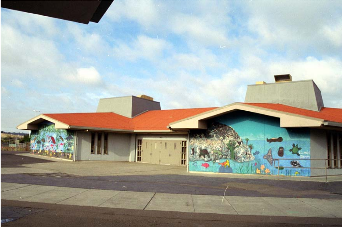
Figure 4: Classroom Building, Unit B, east face
