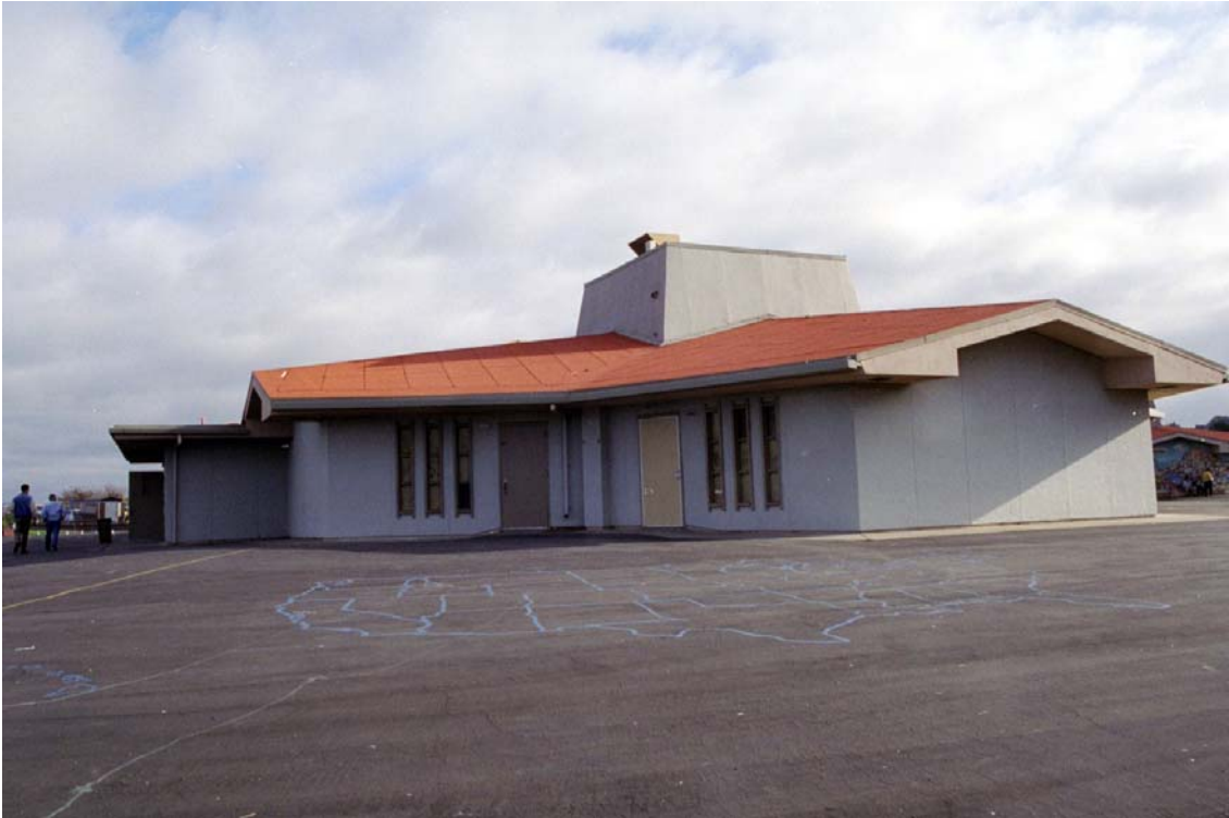
Figure 5: Classroom Building, Unit B, west face
