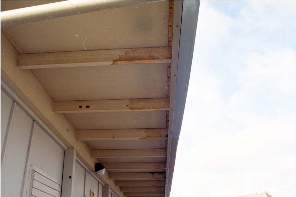
Figure 9: Cafeteria Portable, rusted roof beams
