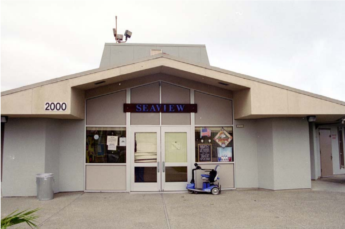
Figure 2: Administration Building, Unit A, main entrance
